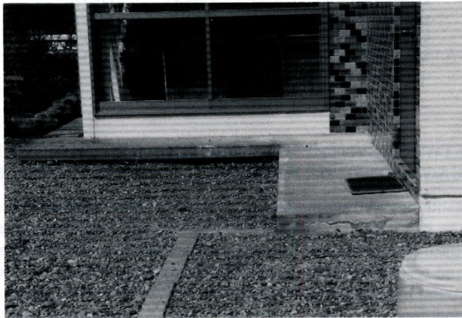
Figure 15. Mihara-3. Dissipation of pore-water pressure built up in the peat layer subjected to the Kushiro earthquake might cause large subsidence measuring over 20 cm at Mihara-3
