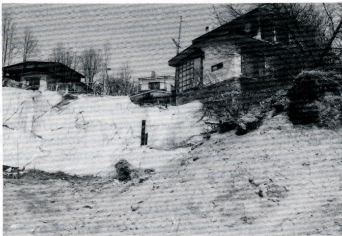
Figure 17. Midorigaoka-6. Large-scale slope failures took place and several houses were destructively damaged at Midorigaoka. Acceleration which reaches 1g was estimated in the analyses at Midorigaoka
