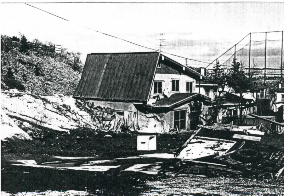
Photo.2 Typical Earthquake damage at Midorigaoka
