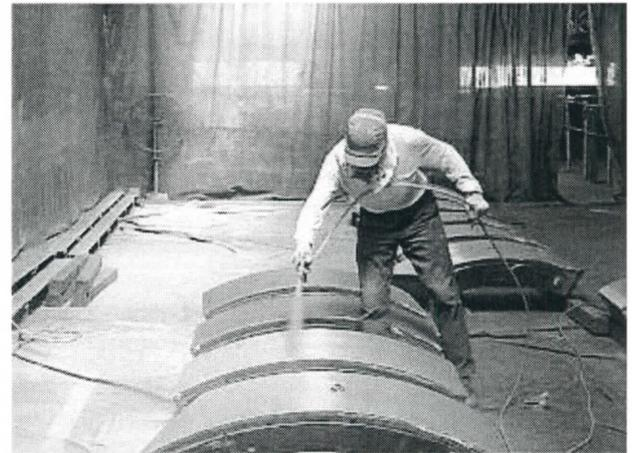
Photo.1 Spray coating on shield segments with slip material.
